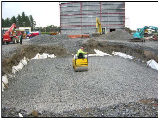
Fig. 2 – Foundation Stone Installed
