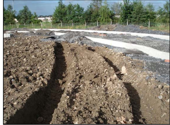
Fig. 14 – Dumper Rutting
