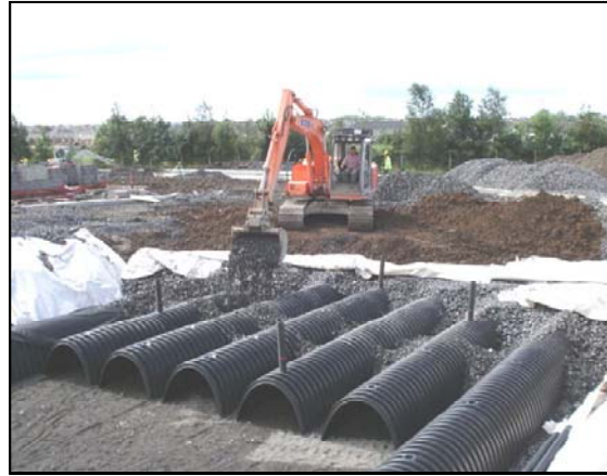
Fig. 9 – Backfilling Stone
