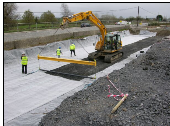
Fig. 1 – Installing GCL Liner
