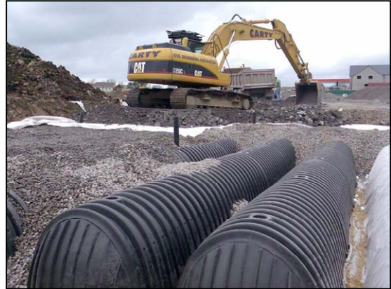
Fig. 11 – Construction Plant over Chambers
