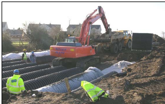
Fig. 16 – Working in Base of Excavation
