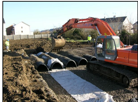
Fig. 15 – Backfilling in Base of Excavation
